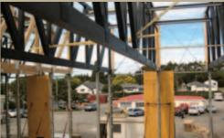
Fabricated from LVL, these giant trusses were fabricated at MTL plant in East Tamaki and transported 650km to Carterton to form the major structural elements for the new events centre. Spanning 25m the deepest of the trusses stands at 4.8m.
